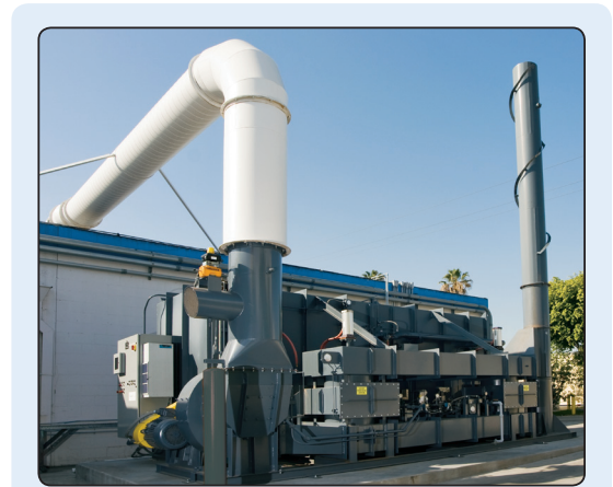
Our California facility takes pride in limiting volatile organic compound (VOC) emissions into the environment. Two regenerative thermo oxidizers are utilized to eliminate 99% of the VOC from our ventilation system before emitting air to the atmosphere.
