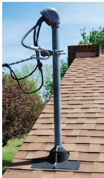
ELECTRICAL MAST ROOF FLASHING
