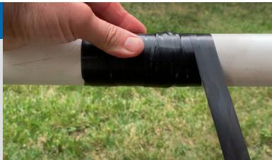
Pipe Repair Wrap can be a long-lasting solution, but it is not intended to be a permanent repair for pressurized applications.
