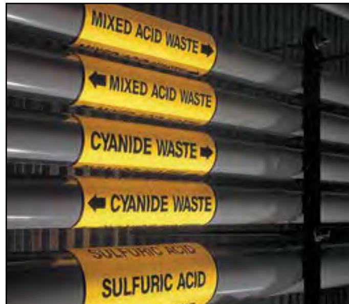
There are several factors that engineers and installers need to take into consideration when constructing thermoplastic piping systems that transport chemicals. Some of these factors include: temperature, pressure, % concentration, location (indoor/outdoor) as well as several others. Follow sound engineering installation and assembly practices as those found in ASME NM-1 and NM-3 (non-metallic codes) as well as ASTM standard assembly practice D2855. Use of P70 primer is required.
