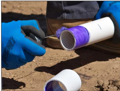
Solvent welding is all about coverage. PVC solvent cement softens the pipe, fills the gap, and creates the bond that holds the system together. Without enough cement, dry spots can form inside the joint, leading to
