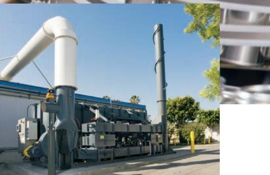
Our California facility takes pride in limiting volatile organic compound (VOC) emissions into the environment. Two regenerative thermo oxidizers are utilized to eliminate 99% of the VOC from our ventilation system before emitting air to the atmosphere.
